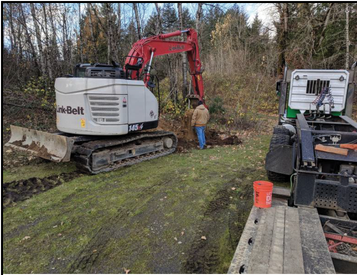
Excavation of test-pit TP-3 looking west
