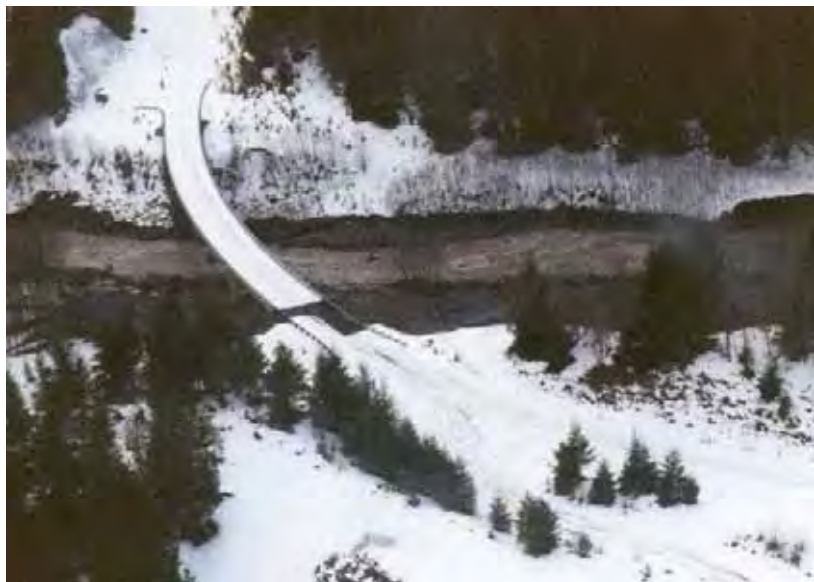
Pine Creek Bridge, 25 Road, 1996, Photograph by David Brown
