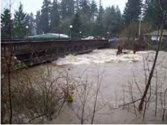
Flood Threat, Rock Creek Bridge, Stevenson Photograph by Eric Hansen
