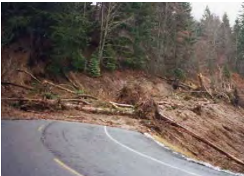
Loop Road Landslide, Stevenson, 1996, Photograph by David Brown
