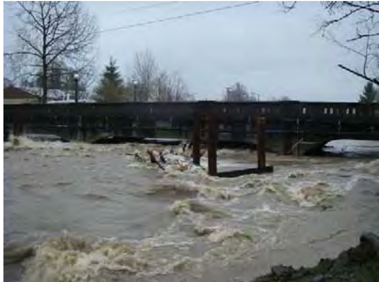
Rock Creek Bridge, 2007, Photograph by Larry Douglass
