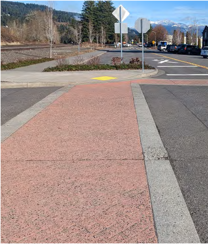
Existing crosswalk improvements for pedestrians.
