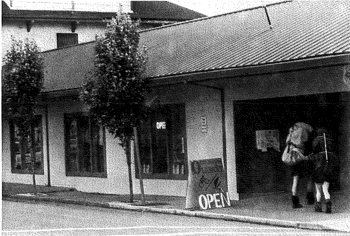
A retail store with stucco walls, wood windows and red corrugated metal roof.
