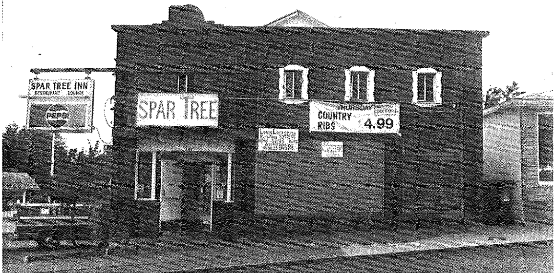
Spar Tree Tavern - one of the best old style storefronts in town. This building is in a highly visual location and could be a real asset to the community if restored.
