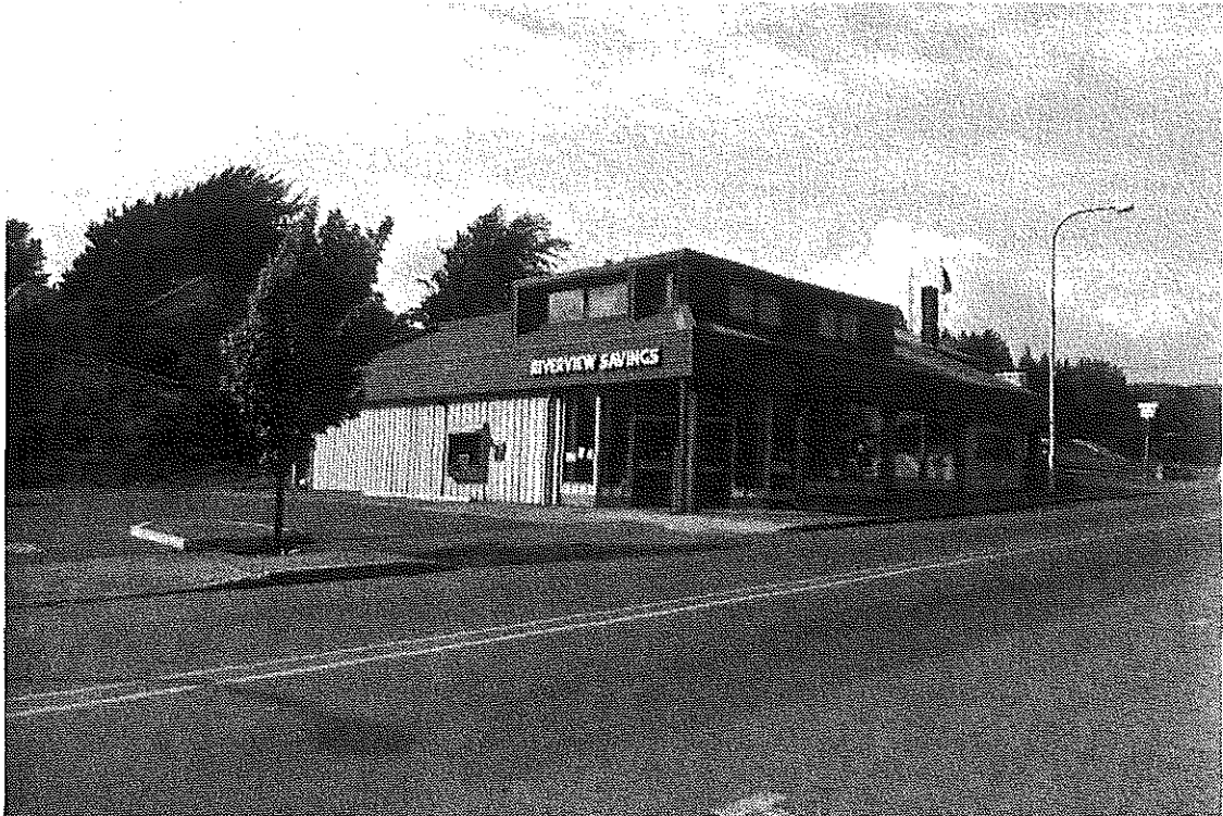
Contemporary savings and loan building facing Second Street. Exterior walls are of stained board siding with a wood shingle accent; the roof is of red corrugated metal.
