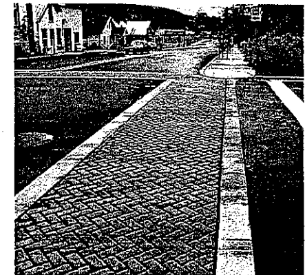
Not Appropriate: Simulated brick or stone from stamped and tinted concrete
