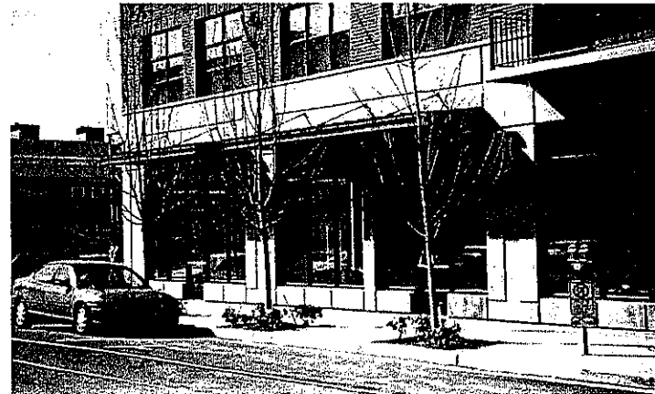
Appropriate: Large retail windows and rain protection
