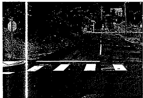
Appropriate: Wide stripes parallel to traffic movements reinforce the zone reserved for pedestrians
