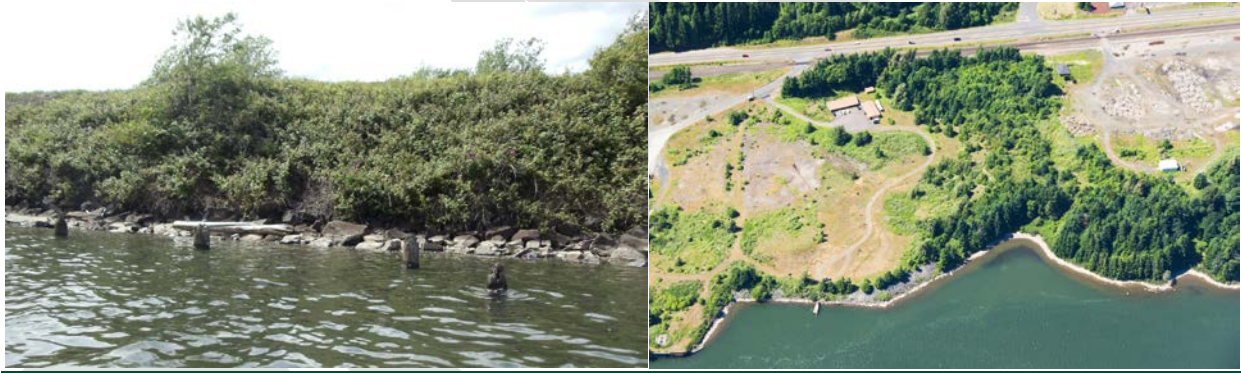
Columbia River Reach 3 Degradation & Restoration Opportunities Derelict piles, riprap slopes & invasive species on the SR 14/BNSF rail road berm. Former industrial development. Photo Credits Ben Shumaker (2013) Washington Department of Ecology (2007).
