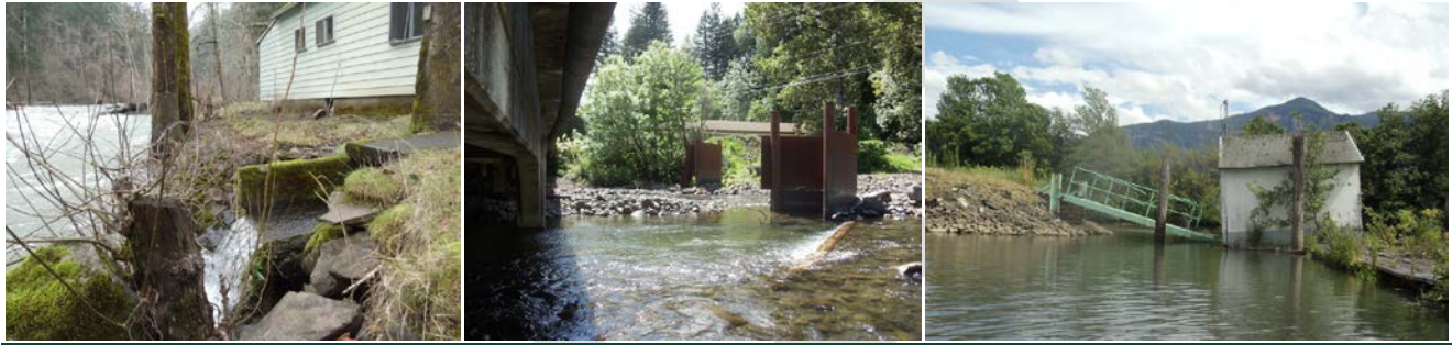
Figure 4.4-3 Potential Restoration Opportunities, Rock Creek Reach 1 Untreated stormwater outfall & abandoned residence. Rock Creek Drive bridge & protective pilings. Abandoned tug boat dock.
