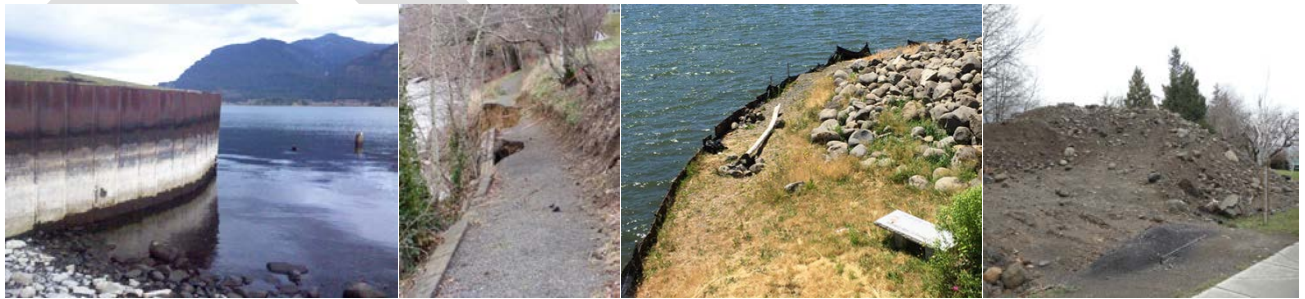
Columbia River Reach 2 Degradation & Restoration Opportunities Sheetpile, active erosion, and staging along the Port of Skamania's Stevenson Shoreline Restoration & Enhancement Project Photo Credits: John McSherry (2010, 2012), Ben Shumaker (2015, 2018).
