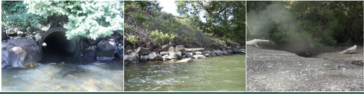
Columbia River Reach 1 Degradation & Restoration Opportunities Differing culvert sizes & elevations, Riprap slopes, and Invasive species along the SR 14/BNSF railroad berm Photo Credits: Ben Shumaker (2013).
