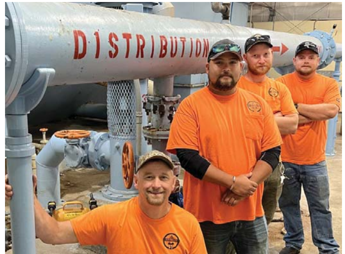
Water Plant Crew
