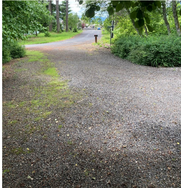
Above – Del Rey (west) looking west
