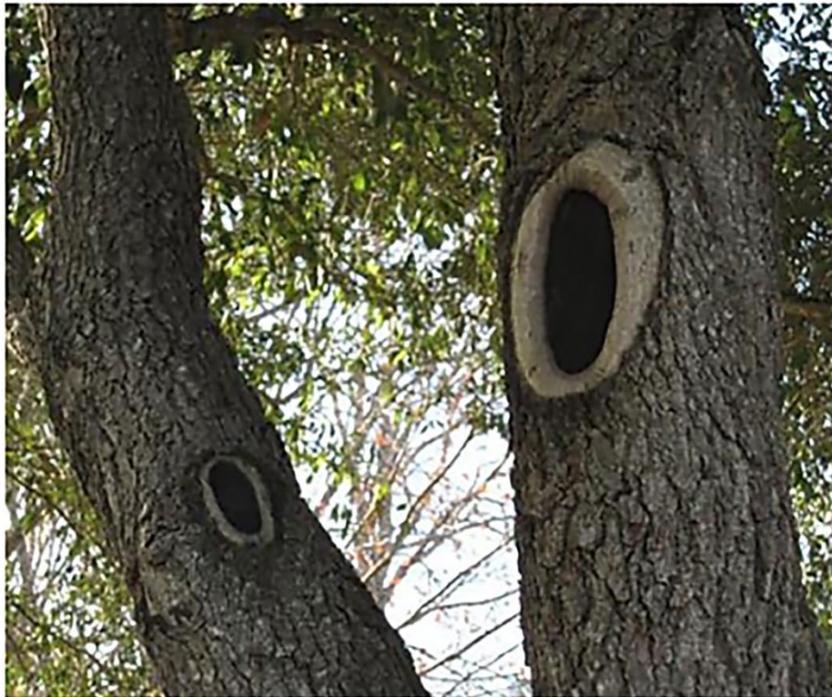
Photo 29. An example of flush cuts. (Not from Stevenson)
