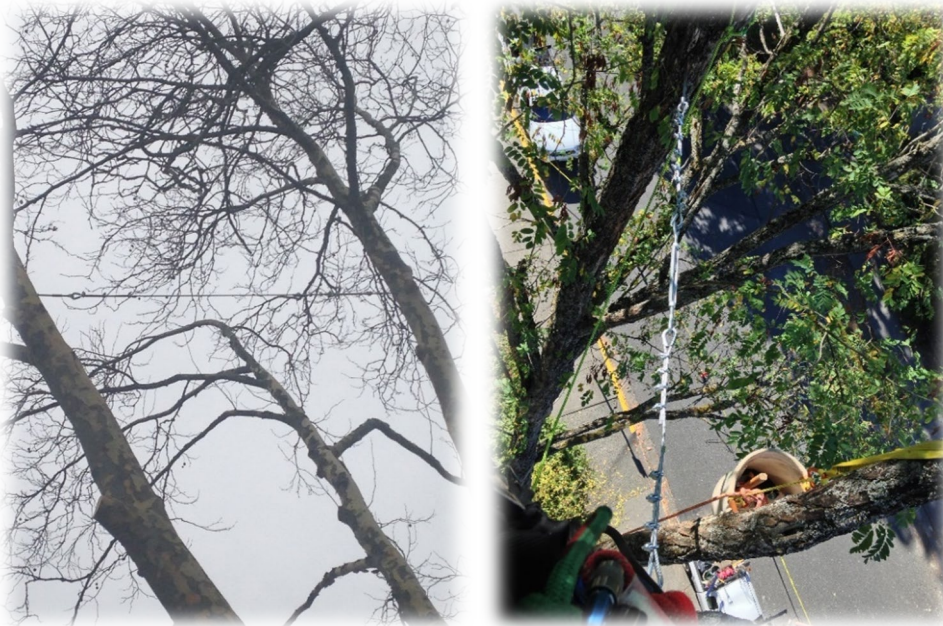
Photo 30, 31 Cabling systems in trees decrease the wind load and movement of large branches.
