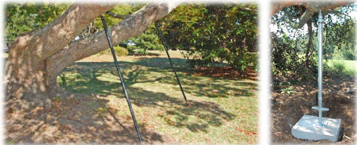
Photo 34,35. Angle Prop system on a leaning tree and an "I" prop showing anchoring and height adjustment
