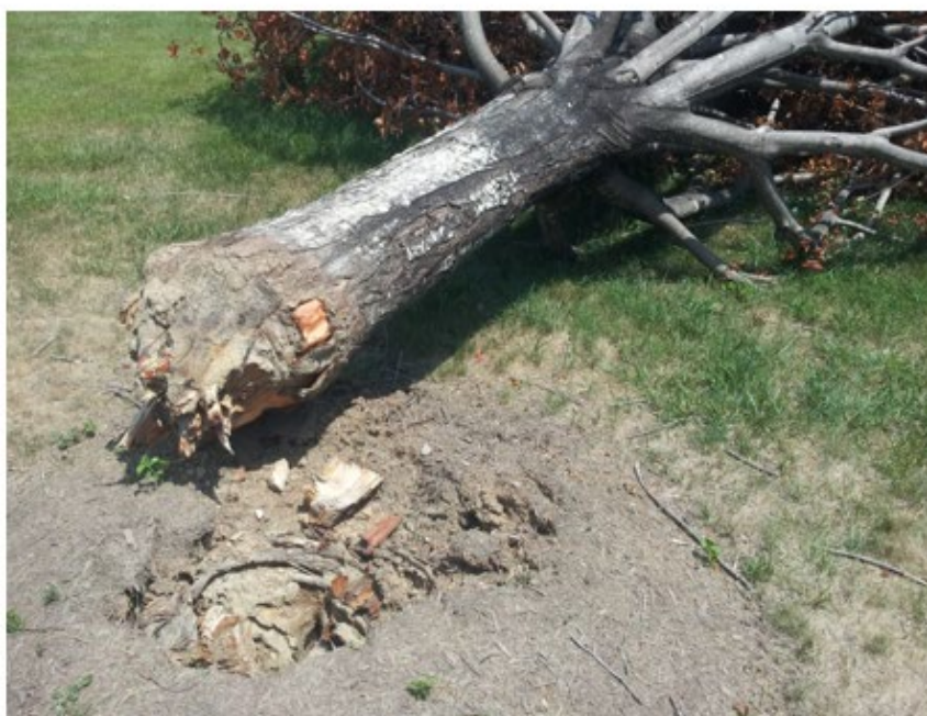
Photo 24. An extreme example of a tree failure brought on by circling/girdling roots. (Not from Stevenson)
